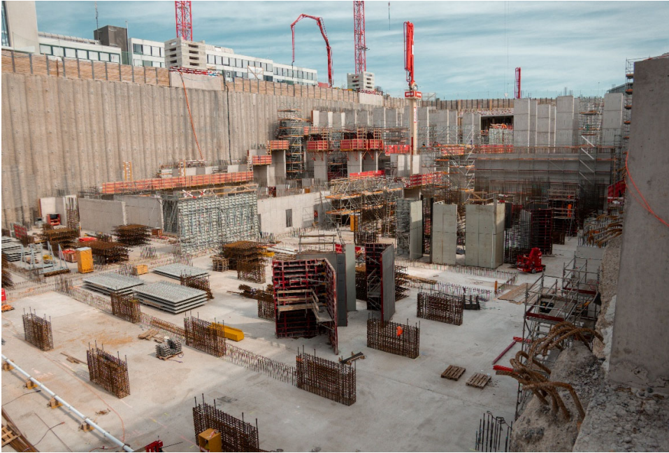
Above: Work on site is proceeding as planned. The excavation work has now been successfully completed. (Photo credit: FlexBase)
